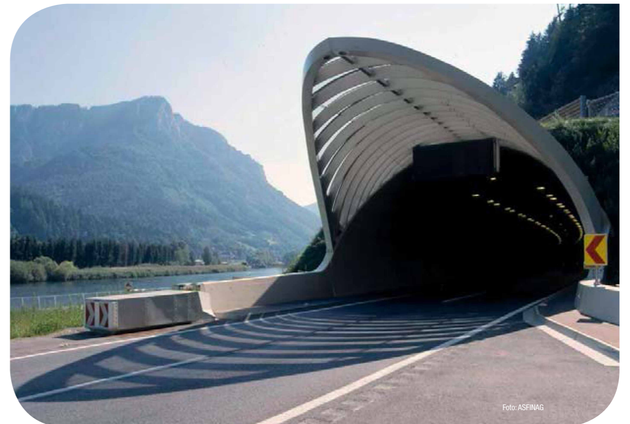
Portal of the tunnel Kirchdorf/Austria where the first pilot system was installed
