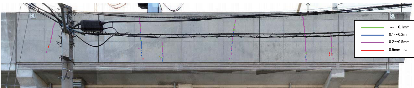
Cracks are automatically detected with size information in different color.
