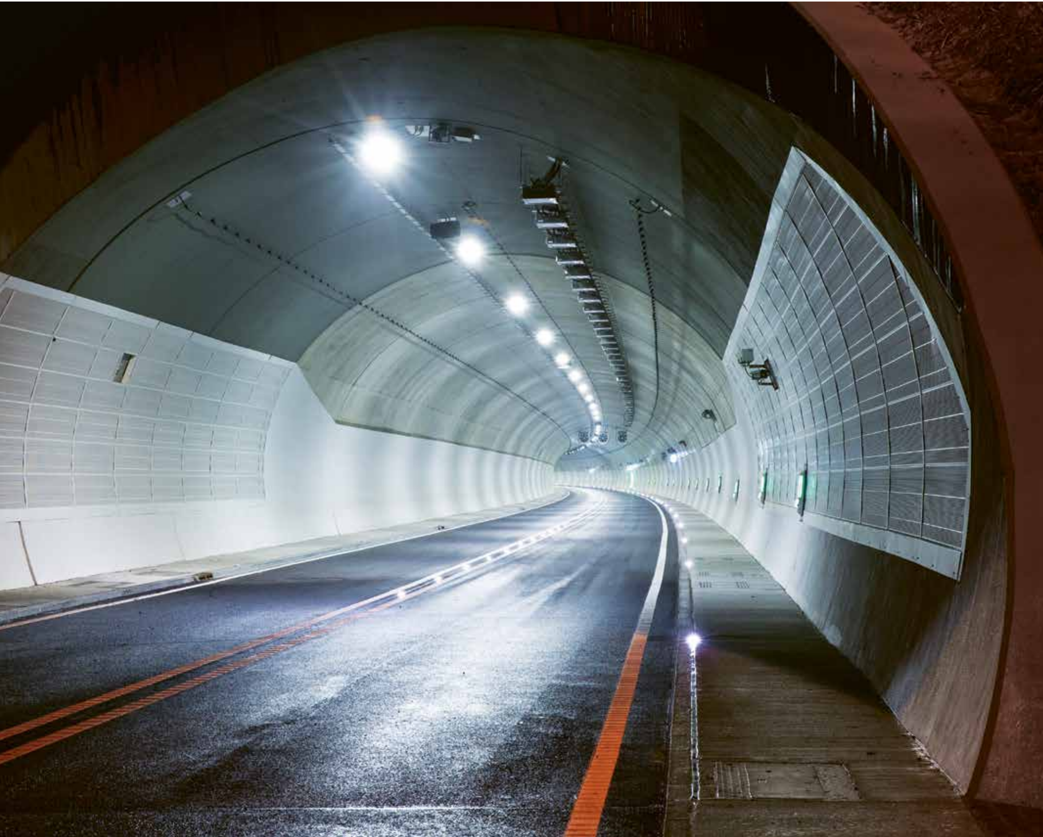
Project: Ettendorf tunnel, Traunstein, Germany Product: Tunnellight TL 33
