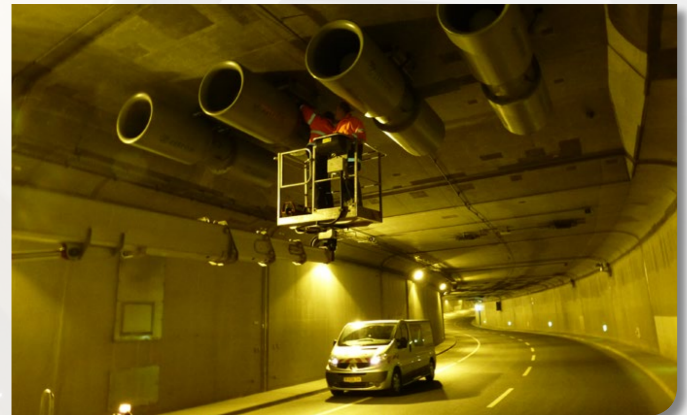
Tunnel Tiergarten - Berlin, Germany
