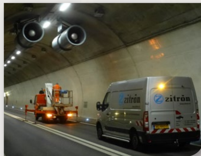
Tunnel Raimeux - Moutier, Switzerland
