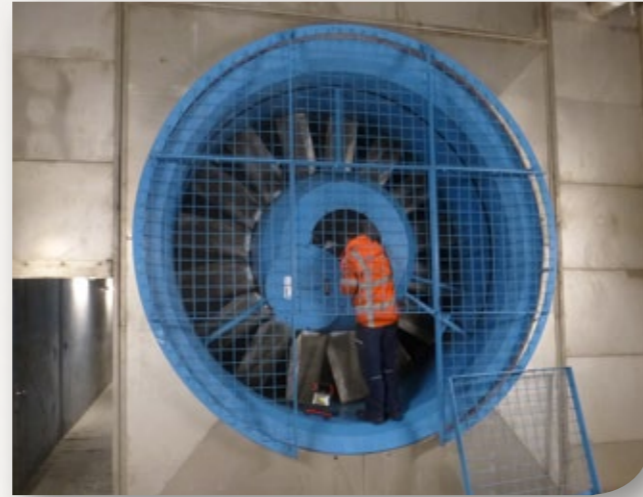
Engelbergbasistunnel - Stuttgart, Germany
