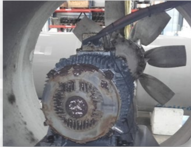
Dismantling of jet fan in Zitron workshop
