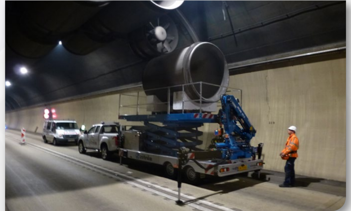
Dismantling of jet fan in the tunnel
