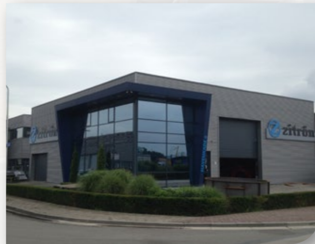
Office location with work shop
