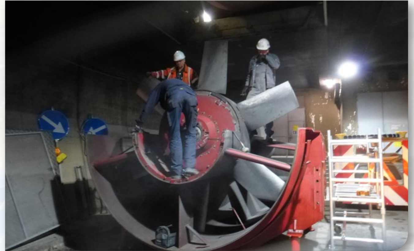
On-site dismantling of fan-motor-unit
