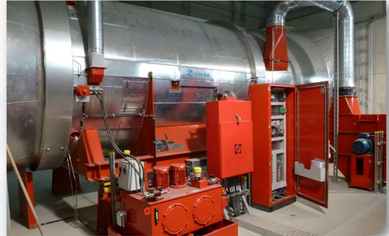
Bosrucktunnel - Arding, Austria
