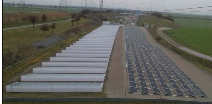
S01 Tunnel Rustenfeld / 130kWp
