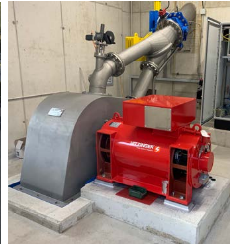
S16 Tunnel Flirsch / 130kWp
