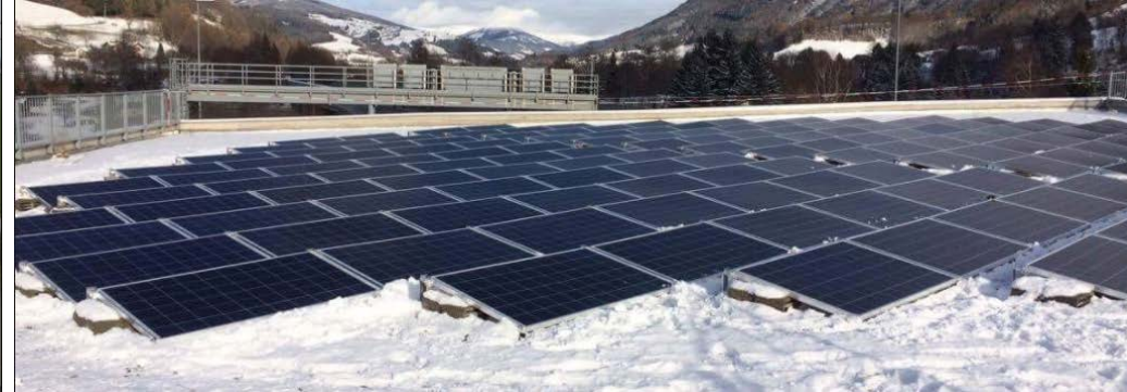
A10 Tunnel Trebesing / 40kWp
