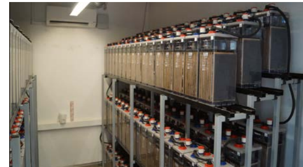
UPS Backup power
