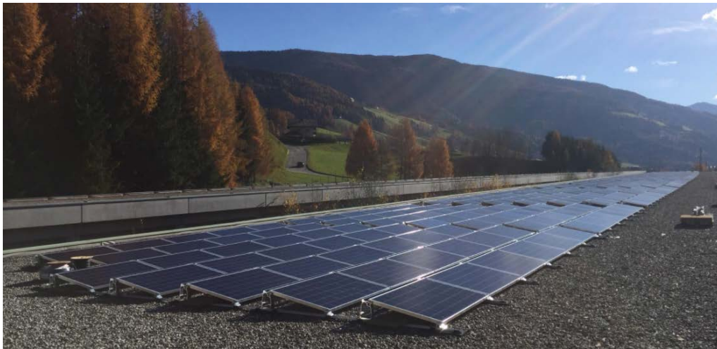
A10 Tunnel Katschberg / 180kWp
