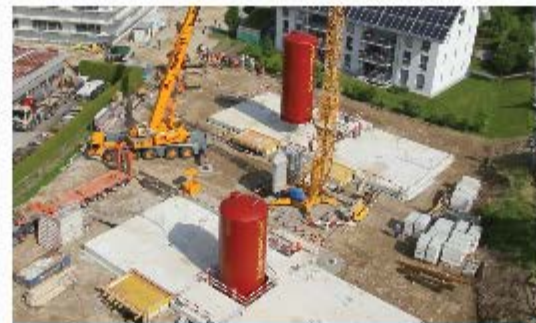
Thermal Energy Storage
