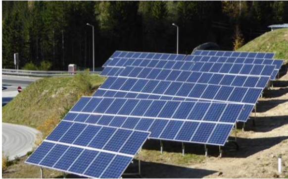
A02 Tunnel Herzogberg / 50kWp
