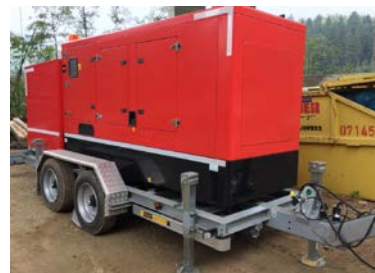
Mobile Diesel Generator
