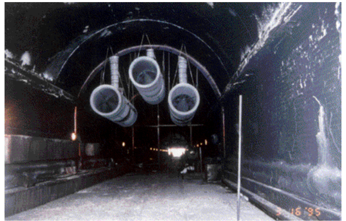
View of jet fan group located south of the fire. Installation typical for all fans (total of 24 fan groups)
