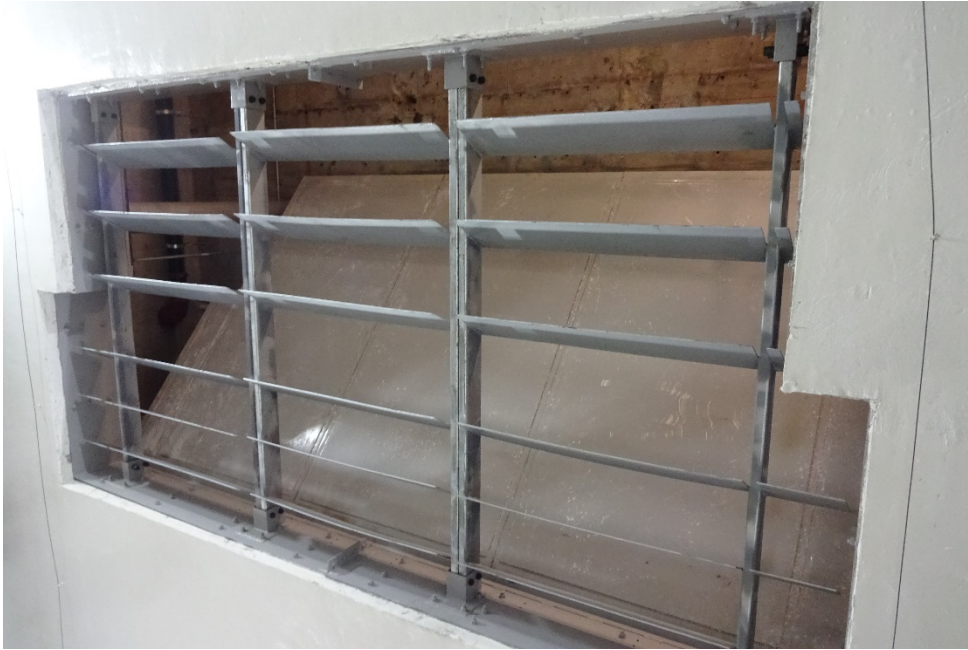
Figure 15: View of installed air vanes from the roadway.
