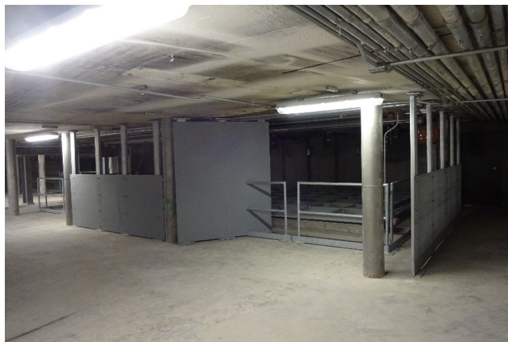
Figure 9: Photos of air baffles
