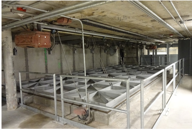
Figure 2: View of damper installation
