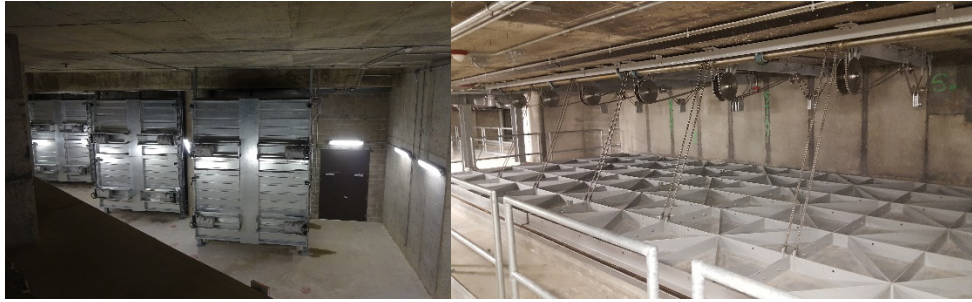
Figure 3: Photos of dampers and installation
