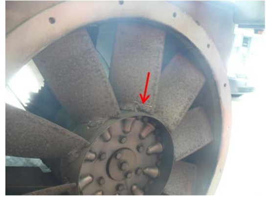
Fig 8: Damaged blade with a partial cut
