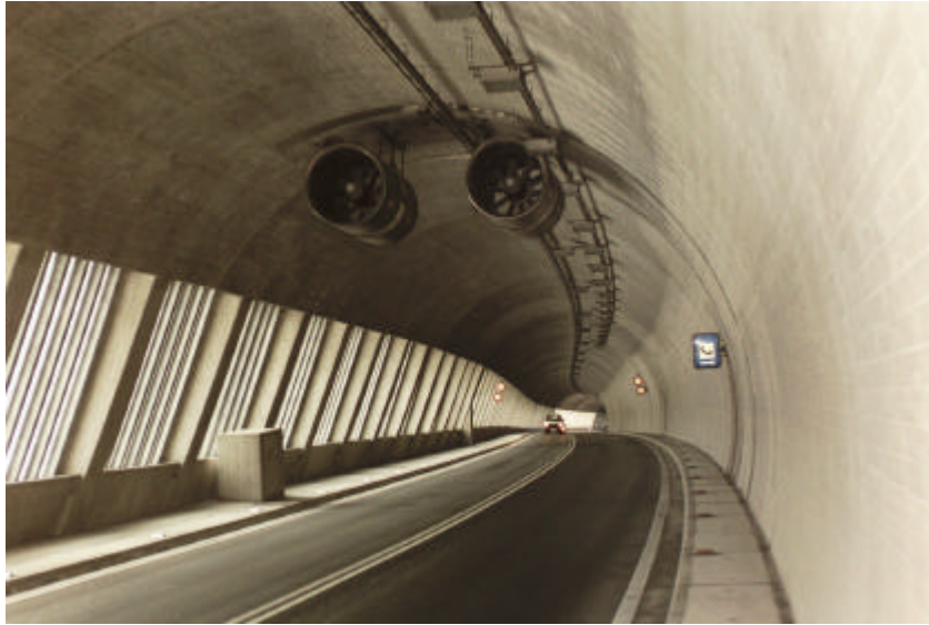
Fig. 1: Jet fan arrangement in enclosed gallery
