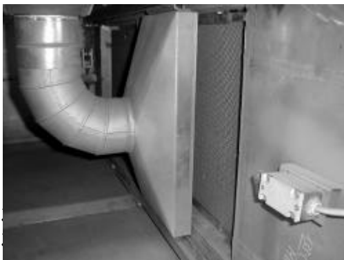
Figure 5 Nozzle for dust collection
