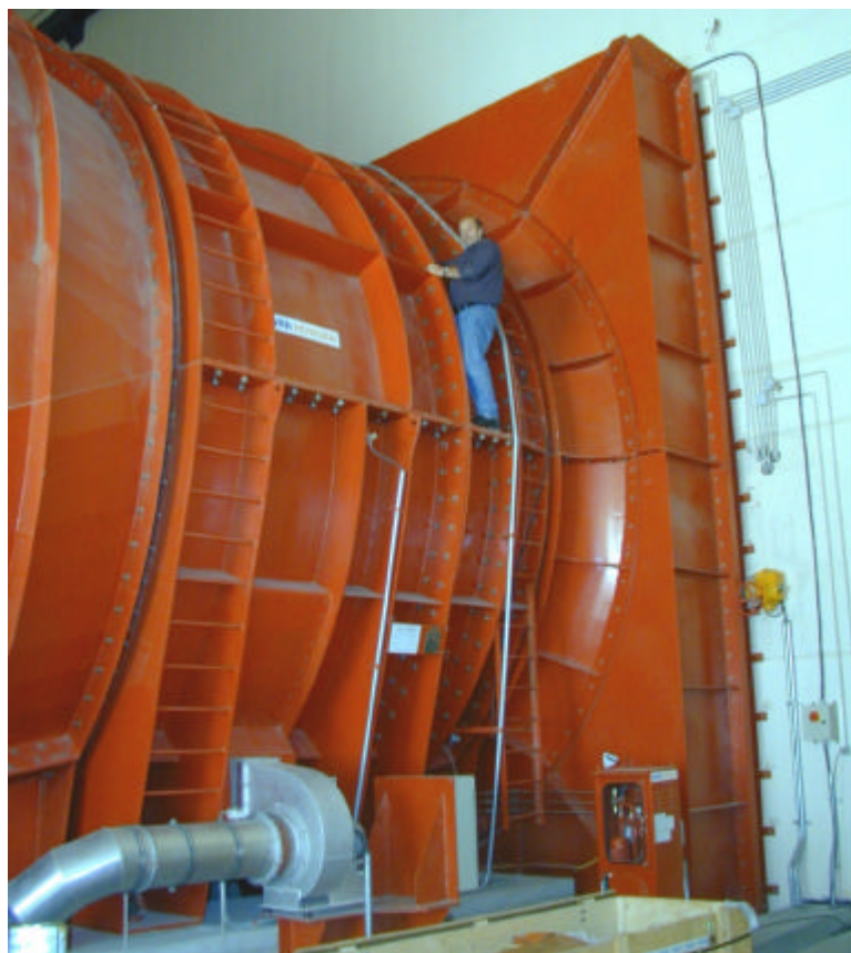
Fig. 7 ST2 Exhaust fan during commissioning
