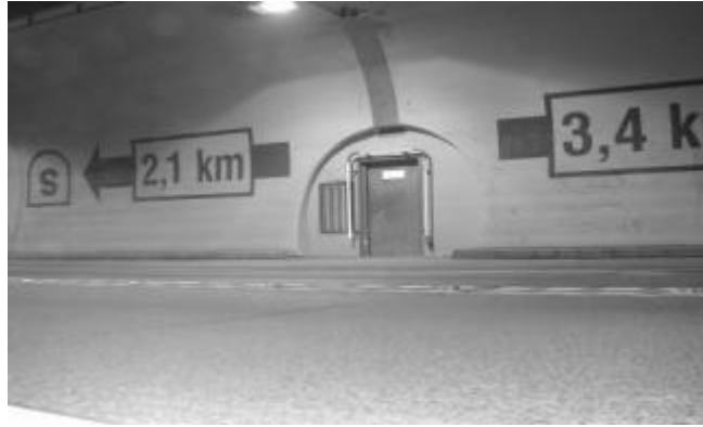
Ill. 6: Breakdown bay with emergency exit leading to the waiting area
