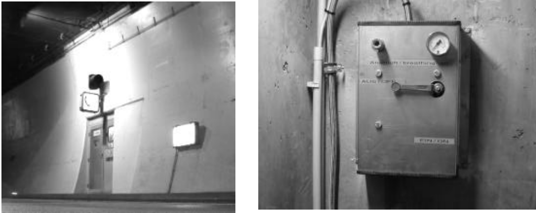
Abb4. SOS niche and fresh air intake ducts
