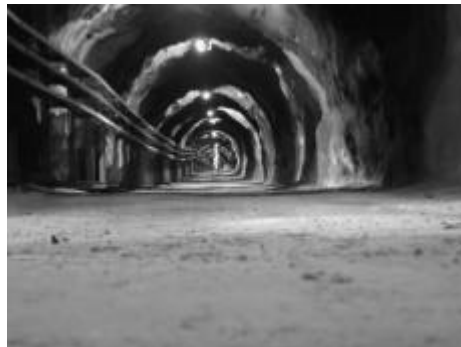
Ill.1: Parallel gallery with cable system
