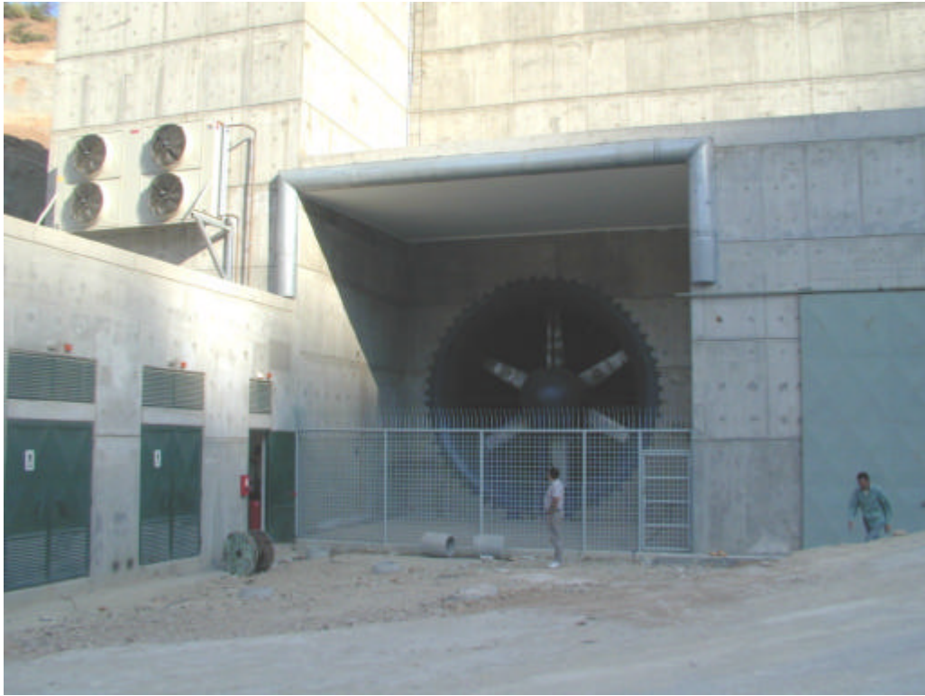
Fig. 4 NT Building supply air intake
