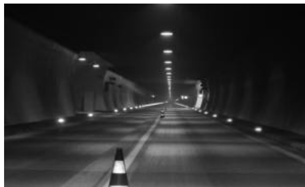
III. 5: LED – reflectors on the kerb
