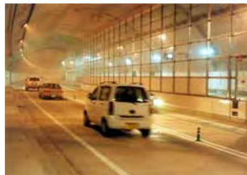
Fig. 3 View from the carriage way
