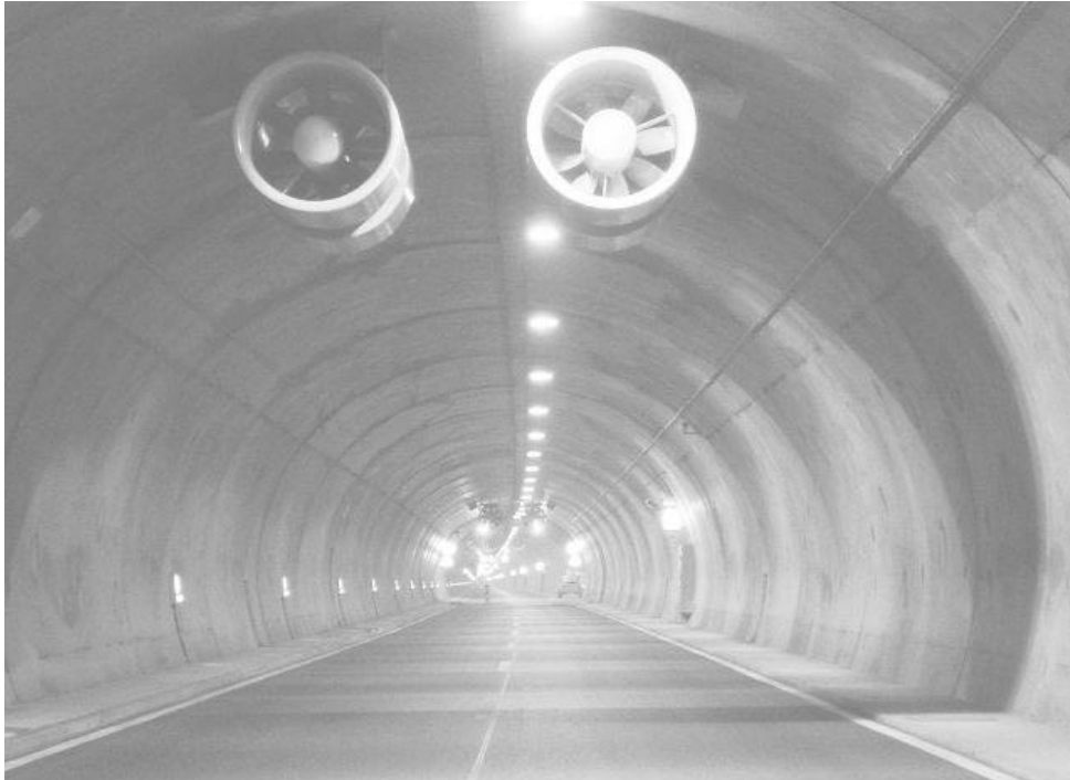
Figure 1: View into the Rennsteig Tunnel with jet fans
