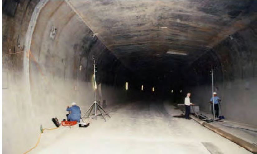
Figure 2: Setting measuring devices for air velocity in the Gotschnatunnel (see chapter 3.3)
