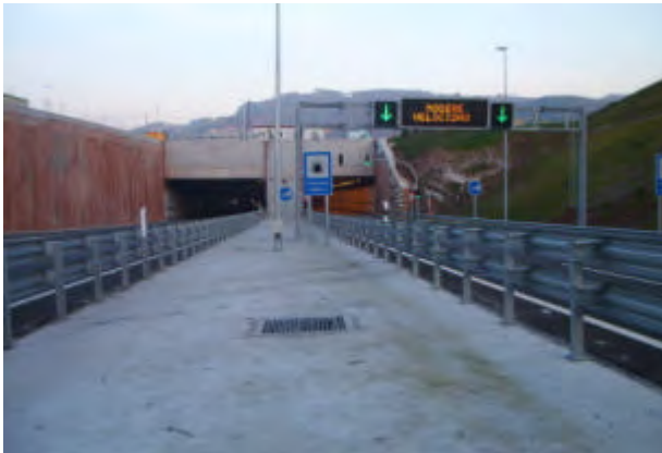
Picture 1: Seen of the portal of the tunnel.
