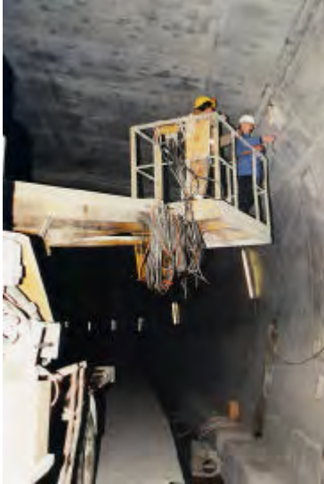
Figur 1: Setting of measuring device for temperature in the Gotschnatunnel
