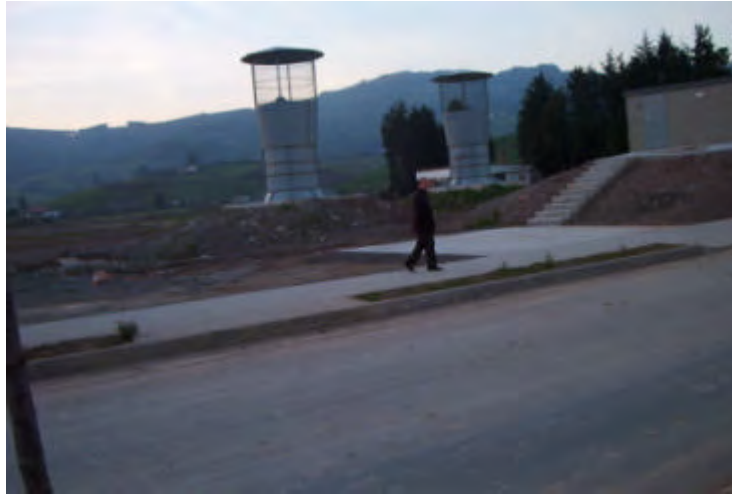
Picture 3: Fans in the exterior of the tunnel
