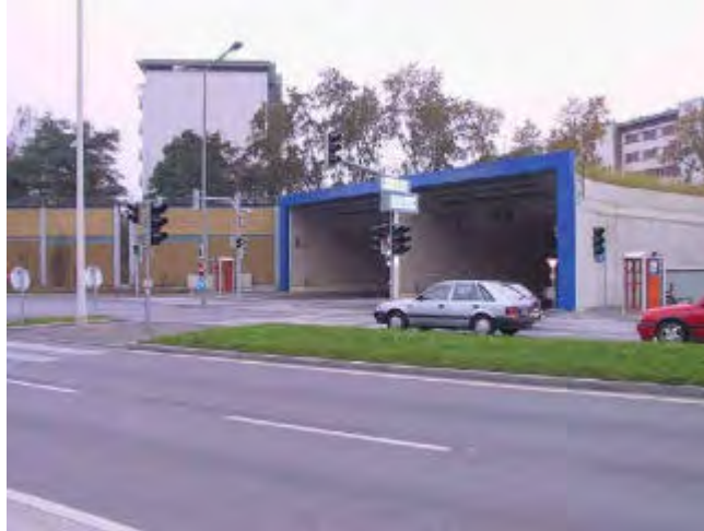
Figure 5: East portal of the “Unterflurtrasse Kalvariengürtel”
