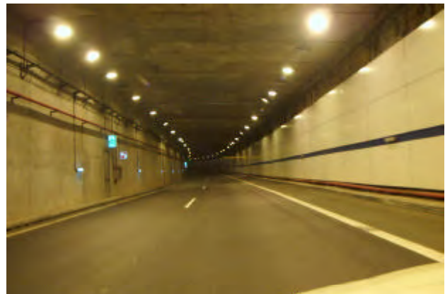
Picture 2: Seen of the interior of the tunnel
