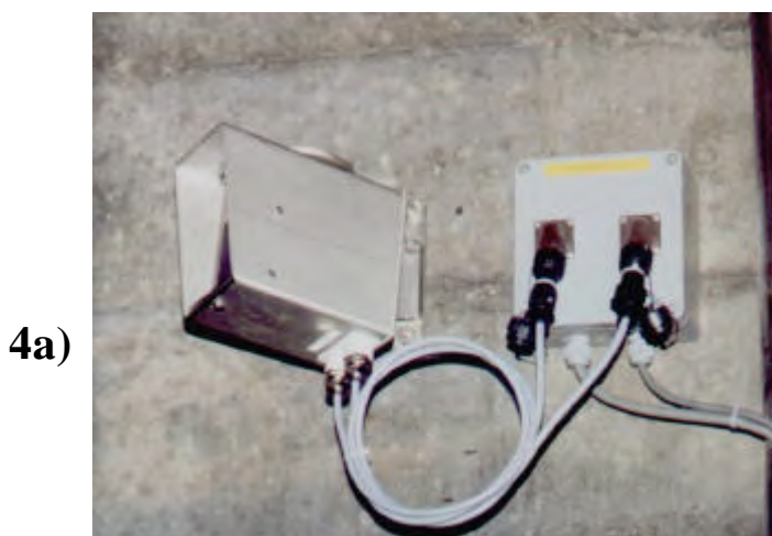
Fig. 4a) An ultrasonic-wave sender and receiver unit for use in road tunnels
