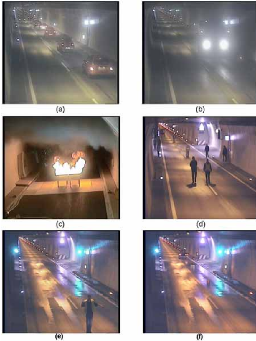
Figure 3: Typical tunnel scenes from our test database: (a) Normal traffic behaviour, (b) Traffic in wrong direction, (c) Fire and smoke, (d) Presence of persons, (e) Presence of persons, (f) Lost cargo. (a-d) dry roadway; (e-f) wet roadway.
