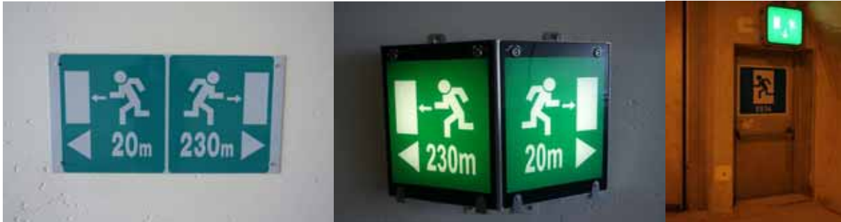
Figure 4: Marking of the escape and emergency services routes
