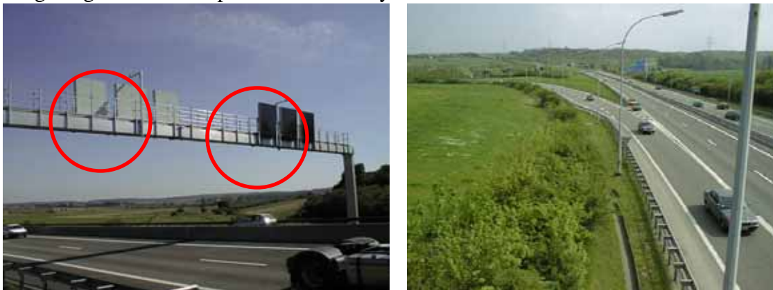
Figures 1 & 2: The installation on the Luxembourg highways with video traffic monitoring connected with Variable Message Signs every 1.5 km has proven to be very effective.
