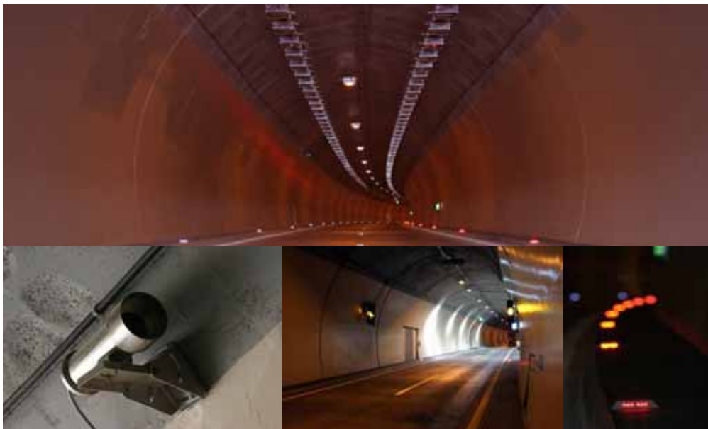
Figure 5: Installations in the tunnel traffic areas
