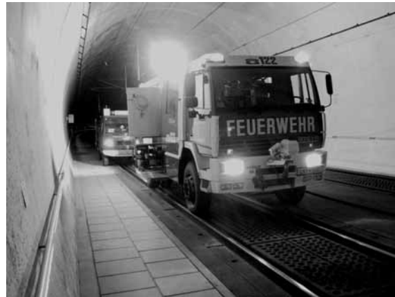
Figure 6: Access area near portal / Accessibility of tunnel by road vehicles
