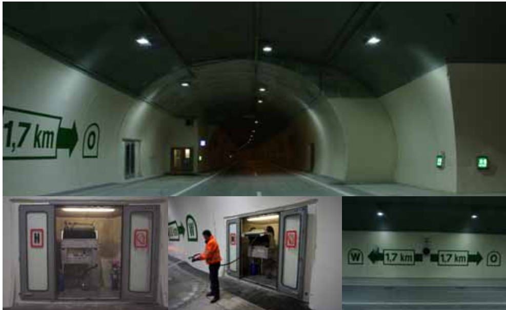
Figure 6: Equipment and installations in the lay-by niches
