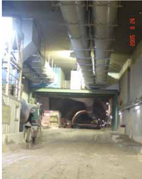
Figure 4: Ventilation and exhaust air fans and air conduits
