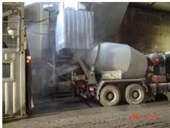
Figure 5: Filling the mixer truck with cement
