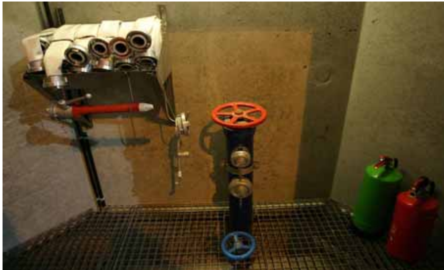
Figure 2: Fire fighting niches for the emergency services
