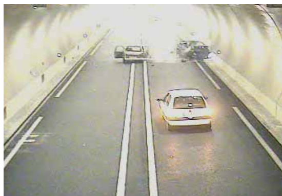
Figure 7: Since the beginning of February 2001, the tunnel of Foix (Ariège - France) is open. With its 2160 metres it constitutes one of the longest tunnels on the French national road network. Right from the beginning, at the time of the risk survey, the commission of security asked for the installation of an incident detection system because of the passage of vehicles transporting dangerous goods.
