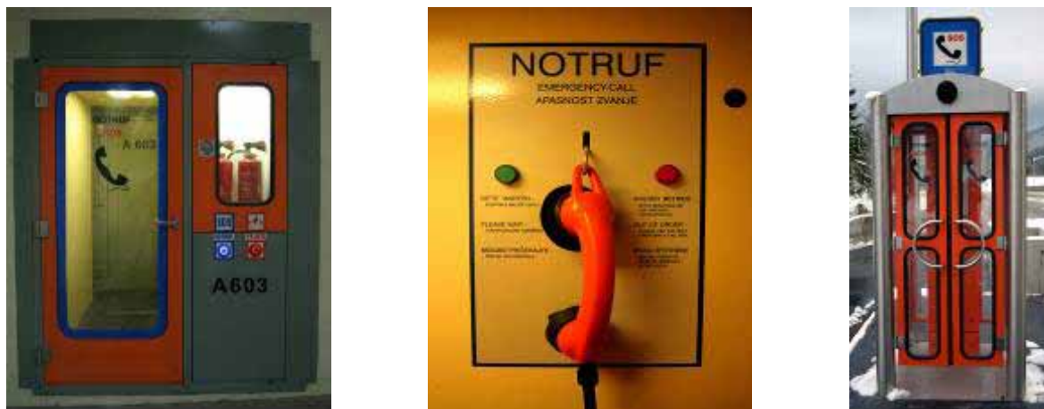
Figure 1: Emergency call installations in the tunnel and in the entrance areas
