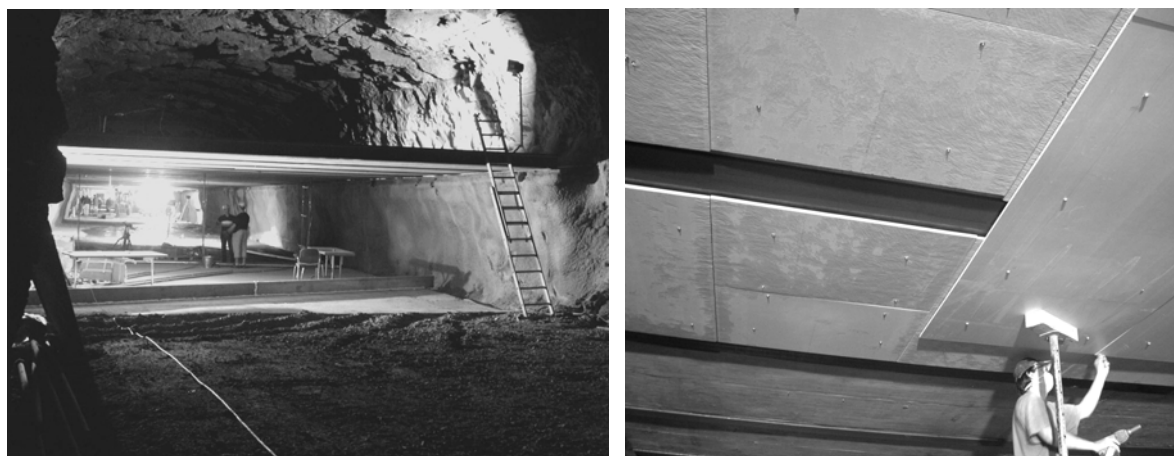
Figure 1: Construction of the concrete ceiling and fire protection in the central fire zone.
