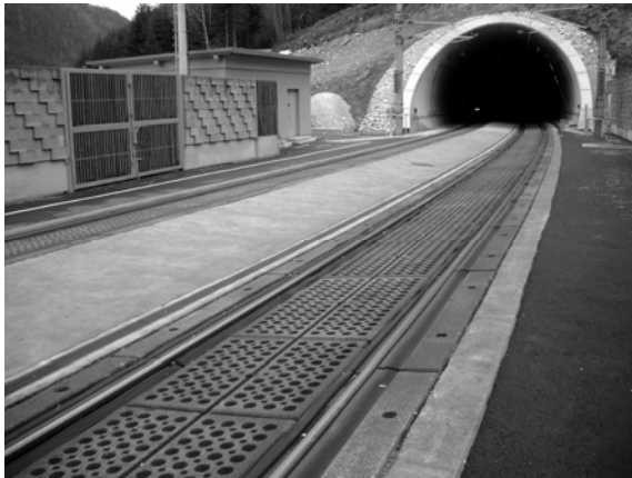
Figure 6: Access area near portal / Accessibility of tunnel by road vehicles
