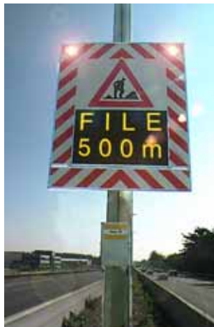
Figure 8: Road works along the E313, Belgium.
