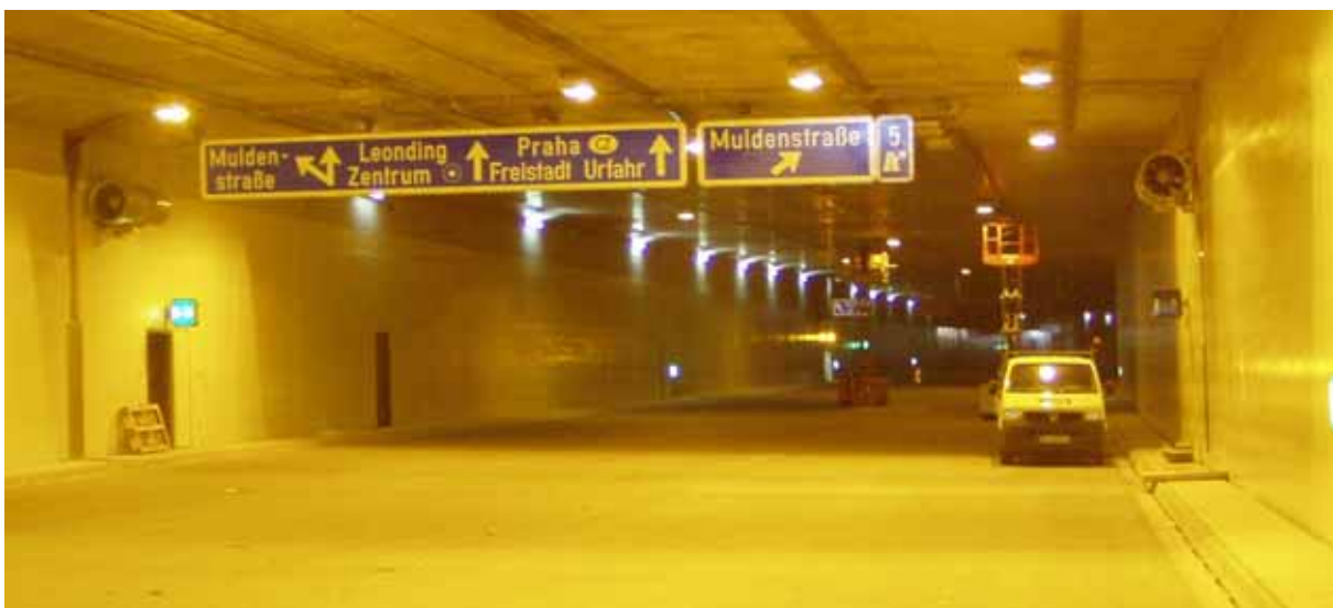
Figure 3: View of the south portal section (zone A and B in Figure 2)
