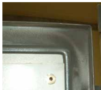
Figure 5: Sealing preventing dust coming into the enclosure (after 15 years tunnel application)
