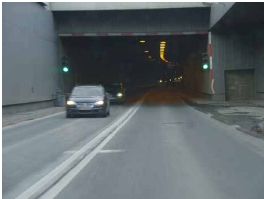
Figure 8: Green lights on both sides of Schmitten Tunnel in bidirectional traffic
