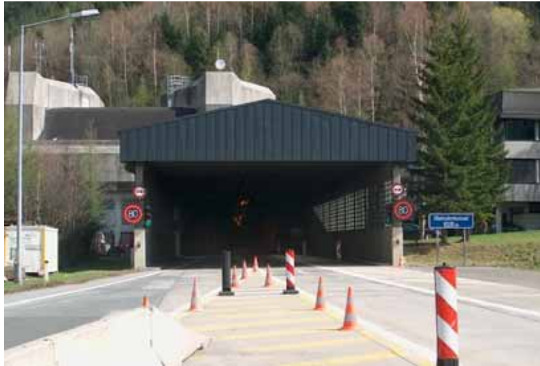
Figure 1: View of the North portal of the Gleinalmtunnel
