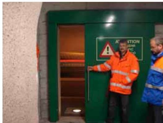
Figure 2: Sliding escape door - view from the side of the safety gallery
