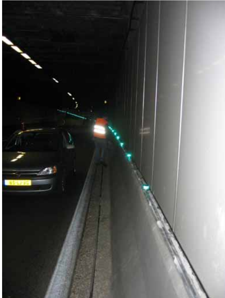
Figure 2: The optical guidance system helps to find the nearest exit - Tunnel A2 Utrecht, NL
