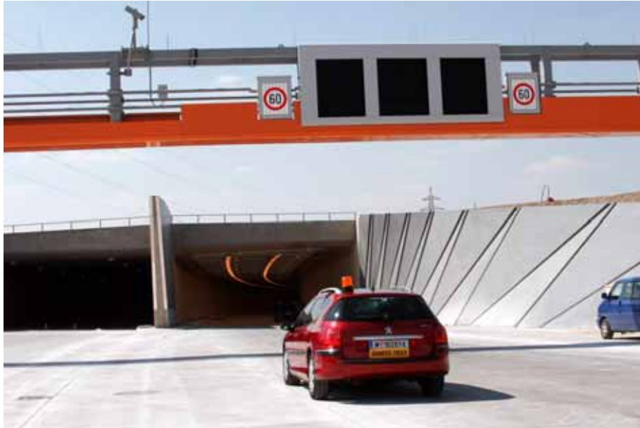
Figure 5: Soft entrances make tunnels safer
