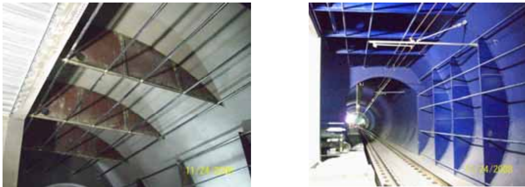
Fig. 1: Baffles as installed in the Beacon Hill Tunnel in Seattle, WA (looking from the tunnel)
