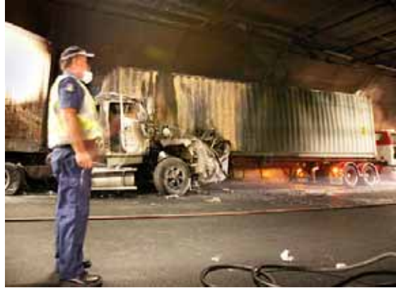
Burnley Tunnel after fire - road surface and tunnel walls and services still intact.
