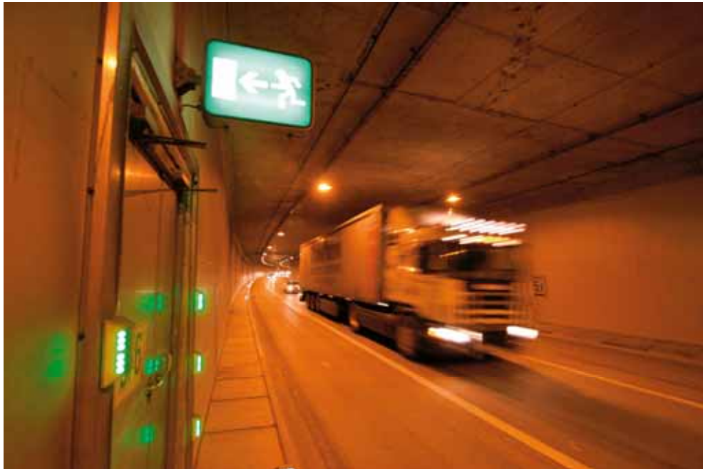
Figure 4: Emergency lane and escape doors reduce the percentage of fear to 50%
