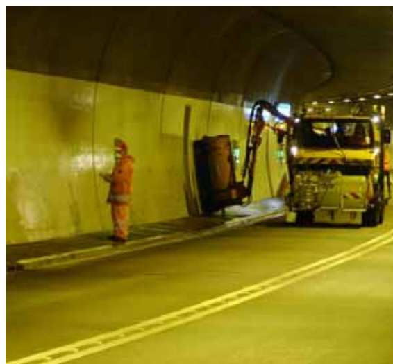
Figure 1: Typical tunnel purification (with friendly acceptance of Andreas Kienzler)
