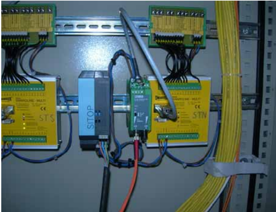
Figure 3: Tunnel Gousselerbiereg, Luxemburg, Multi-system
