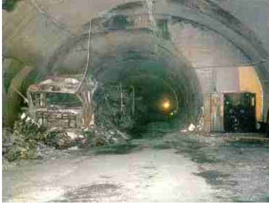
Mont Blanc Tunnel after fire (no suppression system.)
