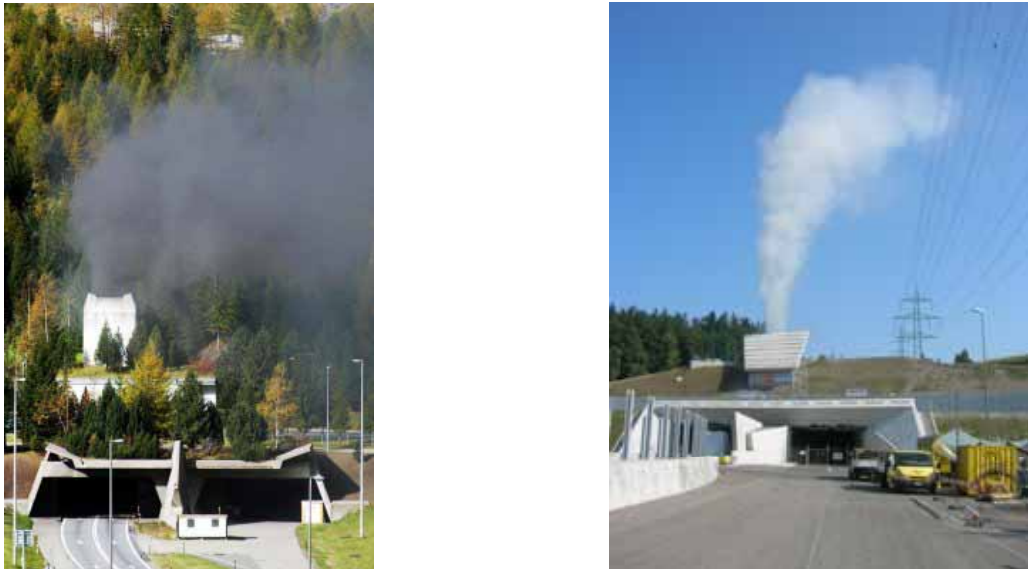
Figure 3: Left: South portal of Gotthard tunnel during the 2001 fire. The distance between portal and stack is 70 m. Right: Test with cold smoke at Islisberg tunnel, jet speed of 20 m/s
