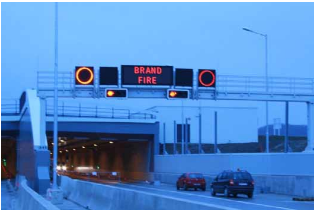
Figure 7: The red lights should flash in case of a traffic stop
