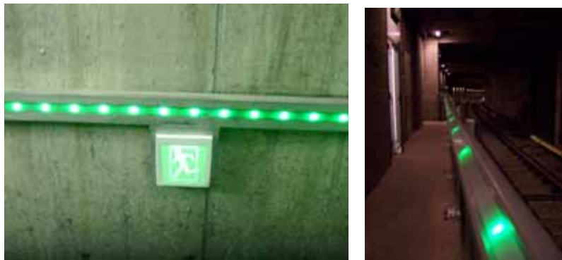
Figures 2: Different installation methods in tunnels. A LED-stripe and symbol panel installed into an aluminum profile on the tunnel wall and into a handrail in a metro tunnel
