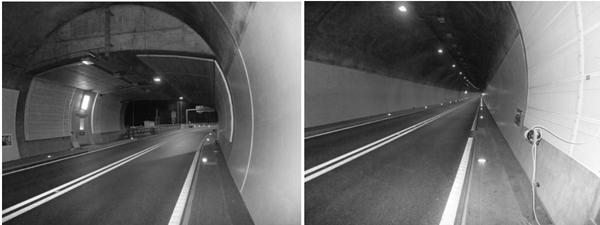
Figure 6: Dosing of tracer gas SF 6 with small ventilators near the north portal in tunnel Flüelen UR.
