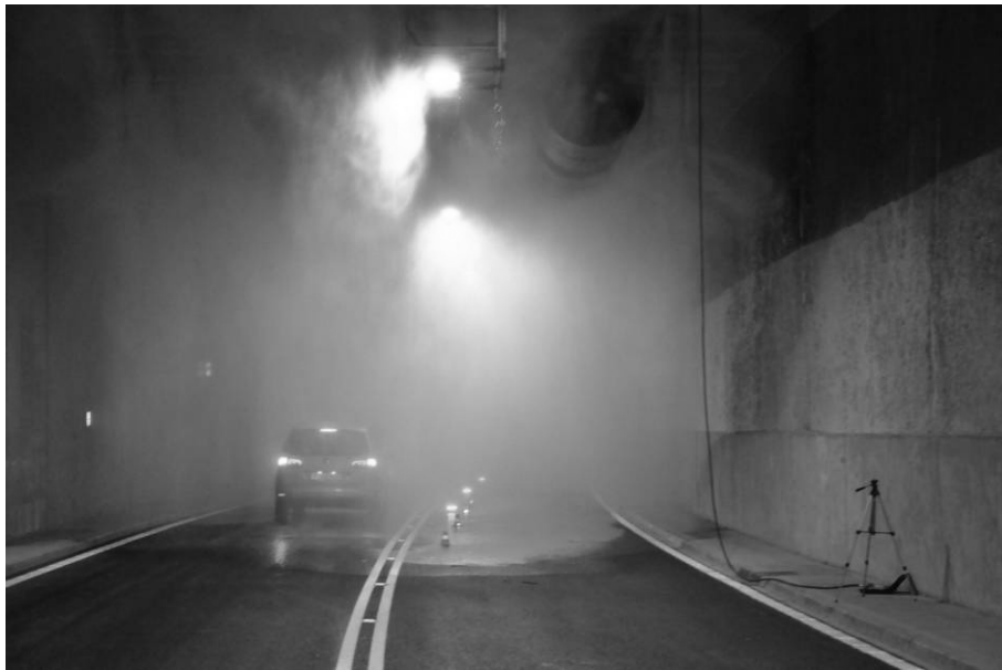
Figure 1: Spray test with a water mist system in the New Tyne Crossing
