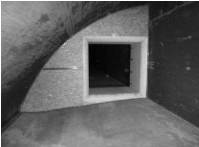
Fig. 8: Measuring nozzle in exhaust duct
