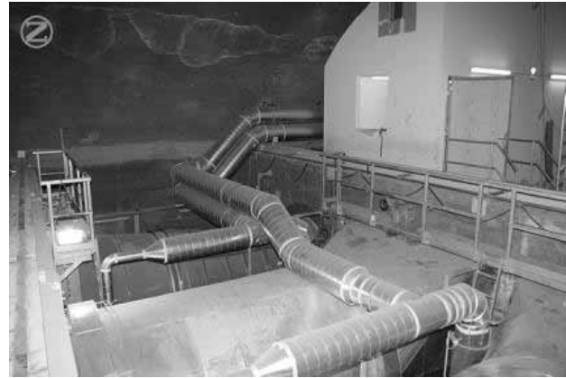
Fig. 7: Auxiliary cooling air ducts
