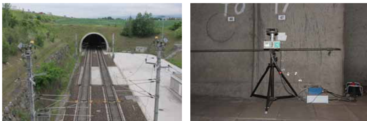
Fig. 2: East portal of Melk tunnel and the measurement setup at km 84.4
