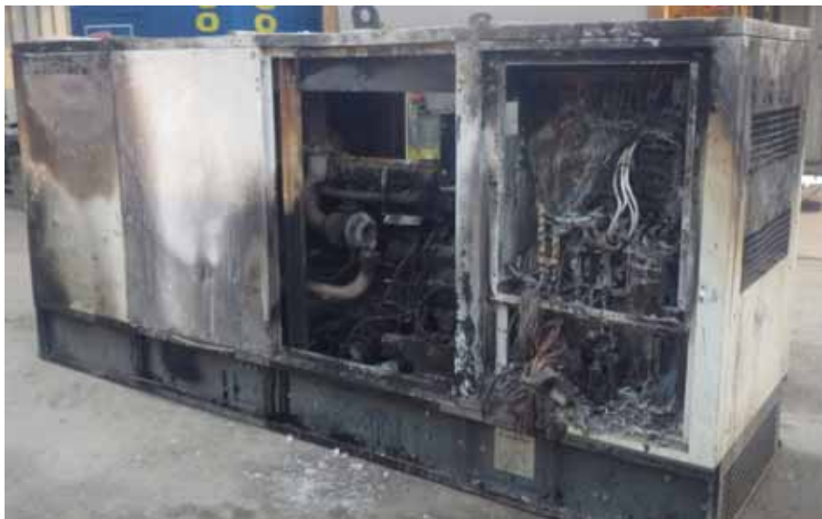
Figure 4: Standby generator after the fire (Source: ARGE KAT2)
