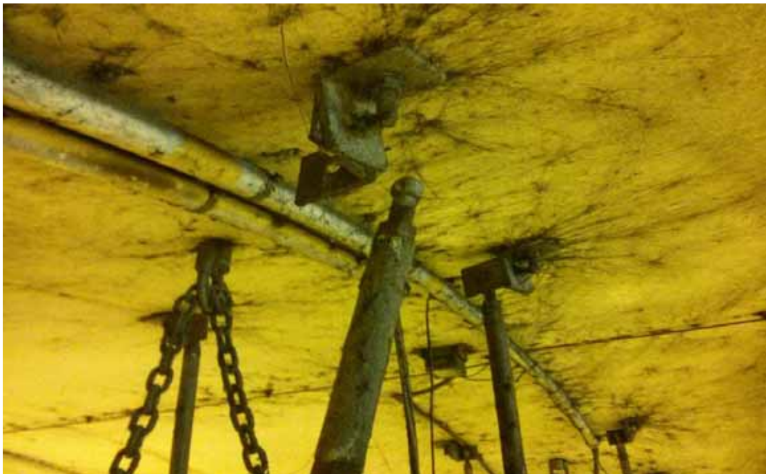
Figure 4: Detail of support break in Lantueno tunnel ceiling
