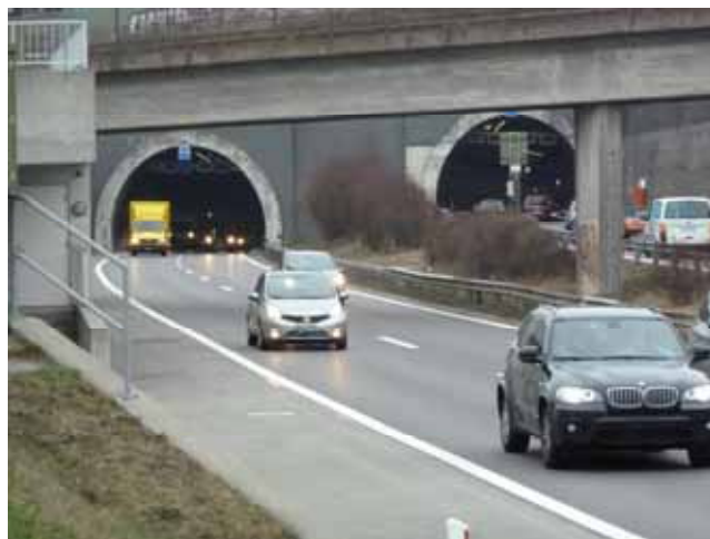
Figure 2: Naturally ventilated tunnel with portals in a deep cut and with potential recirculation of smoke and polluted air
