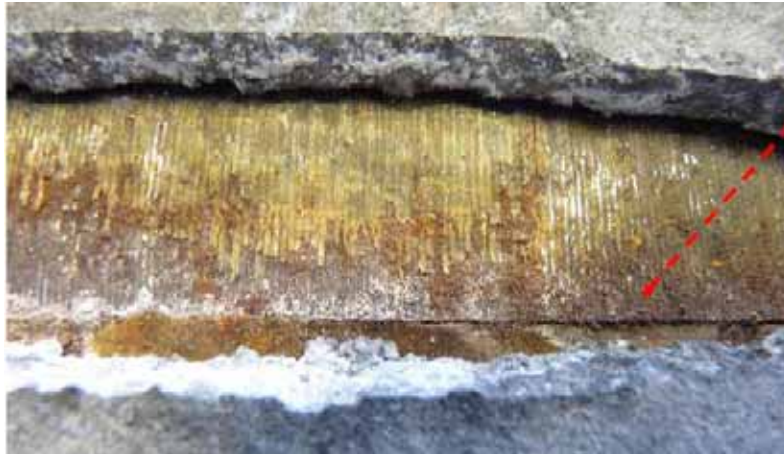
Figure 9: Iron oxides (stator corrosion) of the engine of the fan V5 direction Palencia Lantueno tunnel
