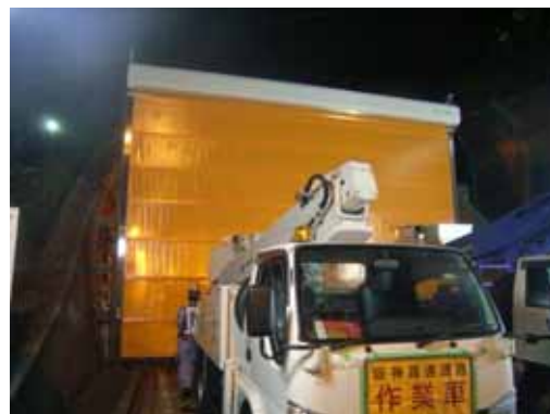
Figure 6: Portal closing device(Close)
