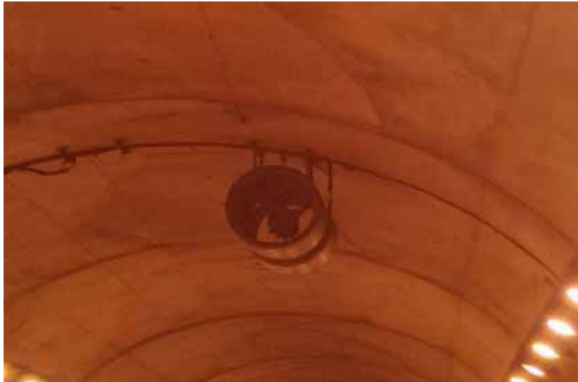
Figure 6: Disassembly of fan in tunnel key of Lantueno tunnel
