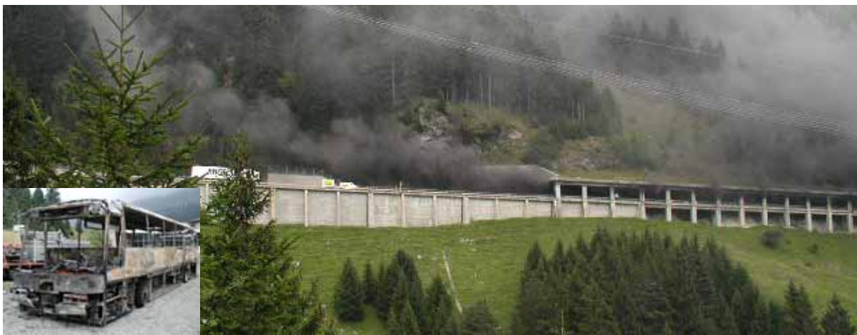
Figure 7: Smoke propagation during a bus full fire (2002). View of the upper gallery portal and image of the bus after the fire in the inlay at the left lower corner.
