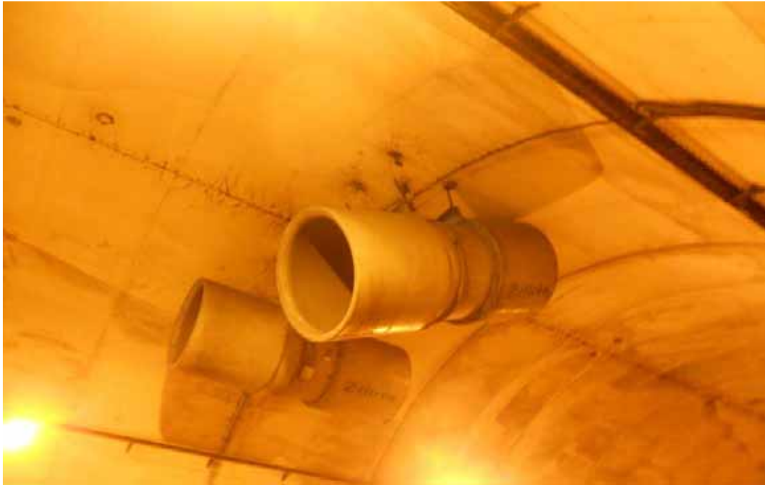
Figure 3: Break of fan support in Lantueno tunnel ceiling
