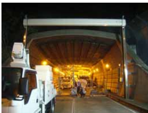
Figure 5: Portal closing device(Open)
