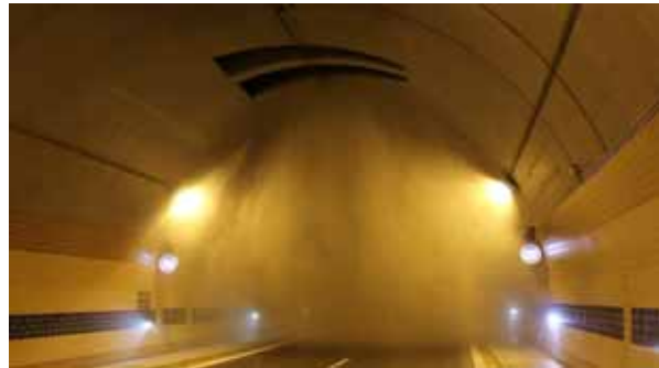
Figure 2: Cold smoke extraction
