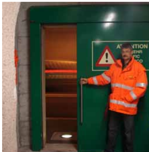
Figure 1: Sliding door seen from pressurized safety tunnel to the deriving space
