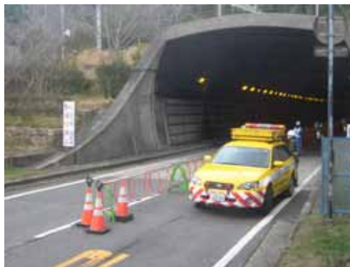
Figure 4: Tunnel portal(Before installation)
