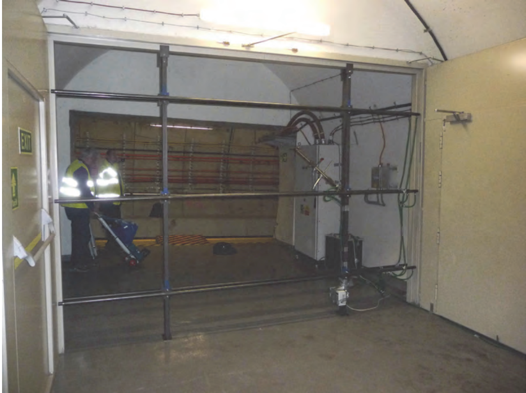
Figure 2: Arrangement of the measurement grid for measuring the dynamic pressure, the installation of propeller and thermo anemometer for measuring the velocity of the air flow within the cross-section of the fire gate in cross passage
