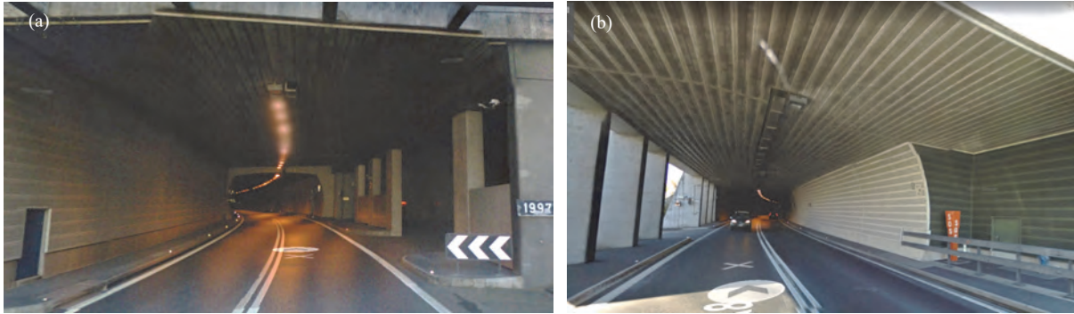
Figure 1: (a) Tunnel portal north, including logistic niche and (b) portal south, including open gallery (Source: Google Maps)
