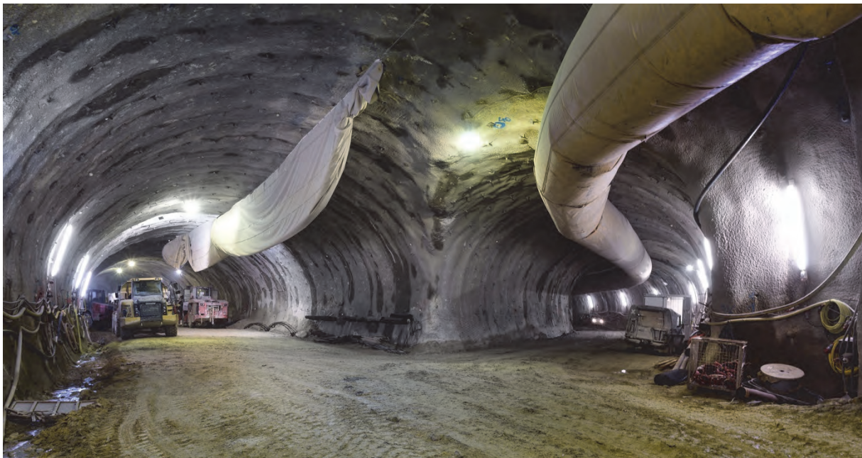
Figure 4: Contract SBT1.1 – Tunnel Gloggnitz: junction at the shaft head area in Göstritz (ÖBB-Infrastruktur AG, Ebner)
