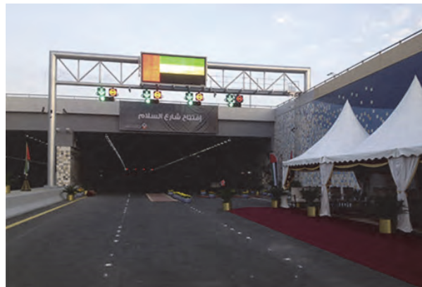
Figure 3: SHEIKH ZAYED TUNNEL Abu Dhabi including control room, United Arab Emirates [2013]
