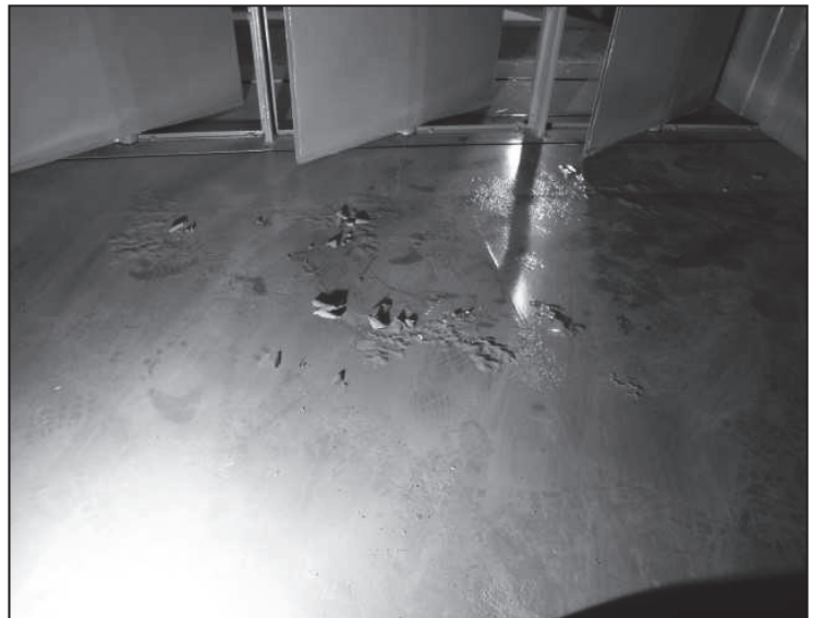
Figure 10: Delamination after treatment
