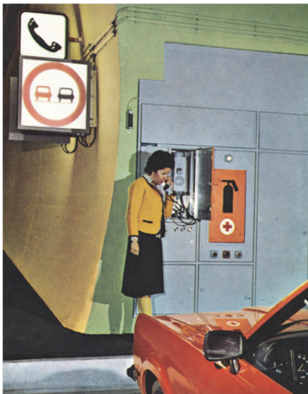
Figure 3: Emergency breakdown bay, Katschberg tunnel, 1975.
