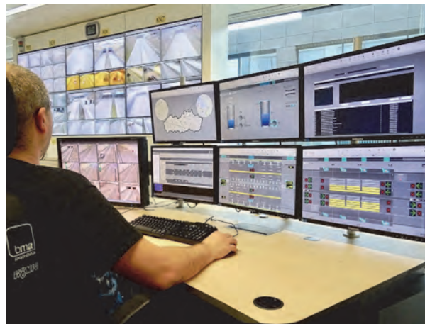
Figure 4: Tunnel management system Vlaamse tunnels, Belgium [2016]
