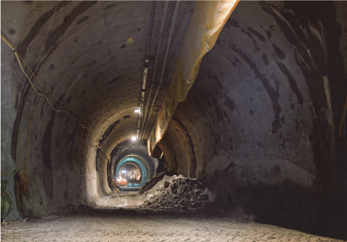
Figure 7: Contract SBT3.1 – Tunnel Grautschenhof: Shaft Sommerau 1, muck removal through shaft (ÖBB-Infrastruktur AG, Ebner)
