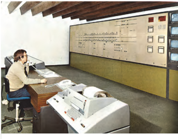
Figure 2: Tunnel control centre room Katschberg-Nord, overall view, 1975.
