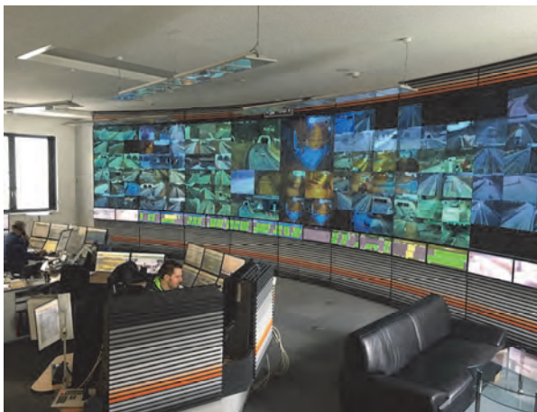
Figure 2: rVMZ Klagenfurt - central control room Carinthia - ZWK [2015]
