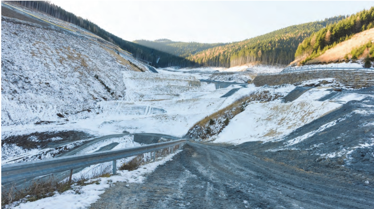
Figure 6: Contract SBT2.1 – Tunnel Fröschnitzgraben: Landfill Longsgraben with the compartment “excavated material” in the foreground and “construction residues” in the background (ÖBB-Infrastruktur AG, Ebner)
