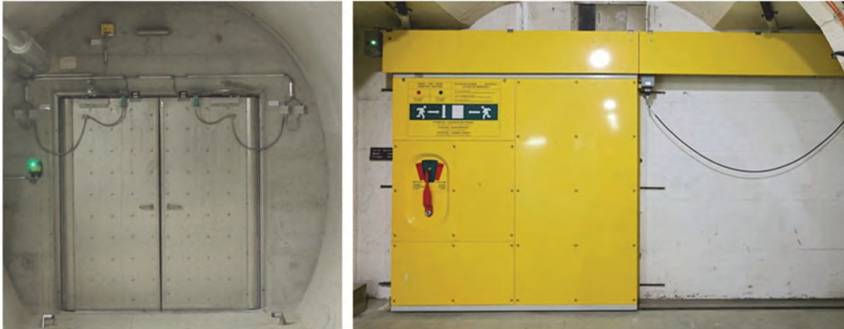
Figure 2: Potential door systems – swing door left, sliding door right
