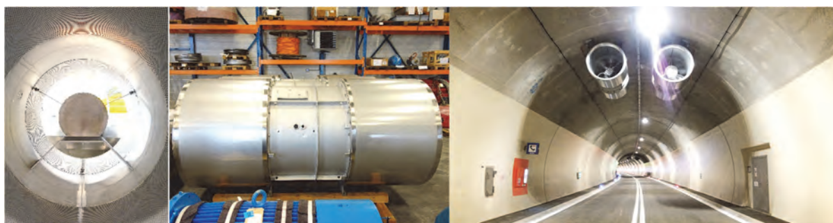
Figure 3: Silencer/fan housing inside (left) and outside (middle), jet fans in Klauser Tunnel (right)
