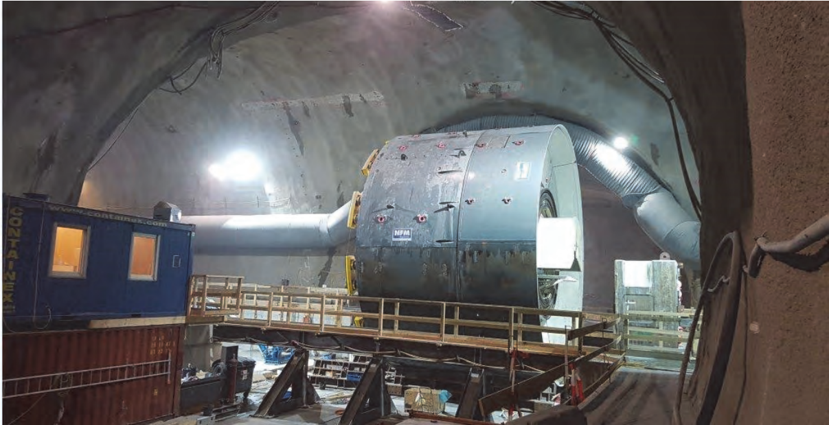
Figure 5: Contract SBT2.1 – Tunnel Fröschnitzgraben: Caverns for construction equipment and the later emergency station
