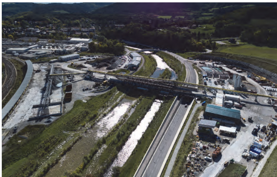
Figure 3: Contract SBT1.1 – Tunnel Gloggnitz: Portal Gloggnitz, Crossing Schwarza (ÖBB-Infrastruktur AG, Ebner)
